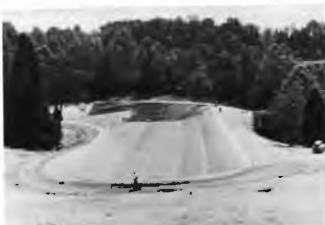
Figure 2 PVC-lined Sediment Storage Area Shown During Construction
