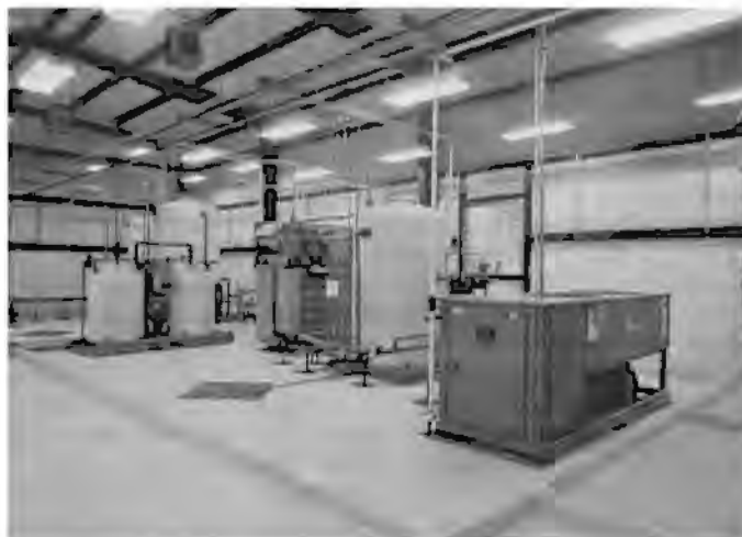
Figure 4 UV/Chemical Oxidation Reactor, Recycle Tank and Chiller
