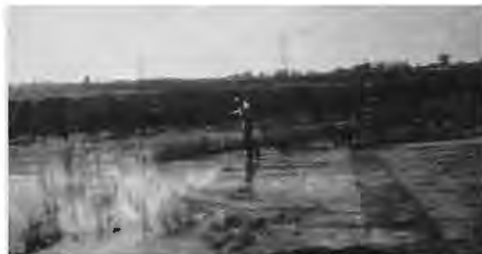
Figure 3 Surveyor Standing on Geogrid Placed on Top of Existing Material which has Consistency of Water
