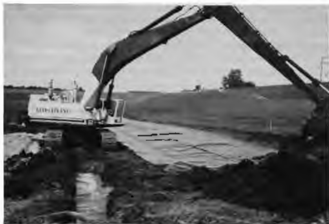
Figure 1 Long-Stick hydraulic Excavator Digging Bio-Polymer Drain
