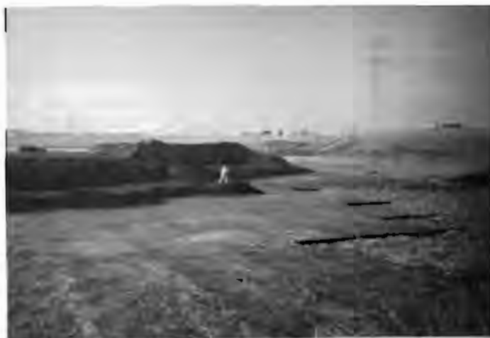
Figure 4 Height of Leading Edge Initial Lift Should be Maintained Relatively Uniform
