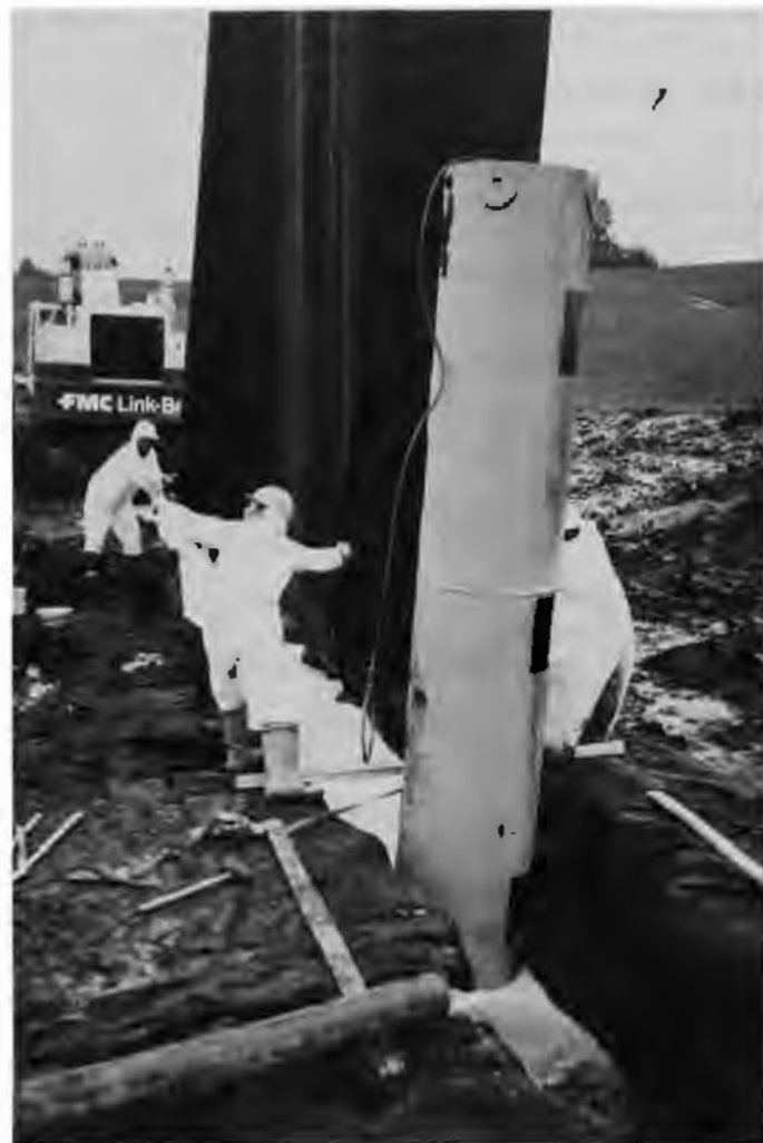
Figure 3 Installation of Geofabric in Bio-Polymer Trench Tremie Pipe in Foreground
