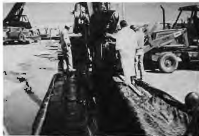
Figure 4 Pipelayer Machine Placing Flexible Perforated Pipe in Bio-Polymer Trench
