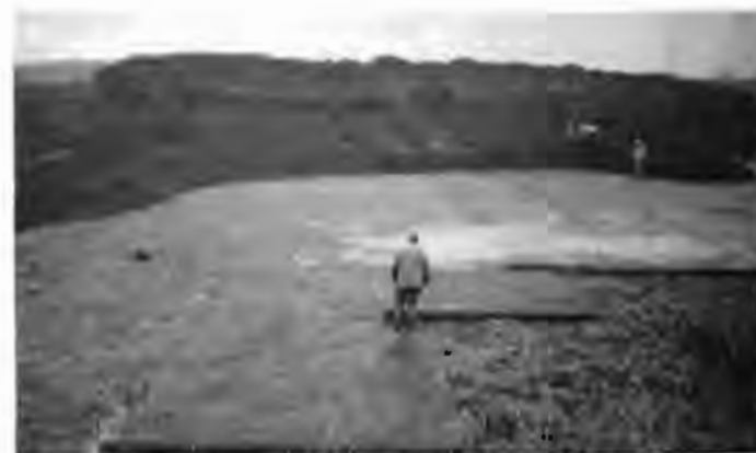
Figure 5 Geogrids Do Not Need to be Anchored at Roll Ends
