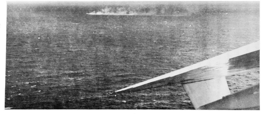
Figure V-4 Plume of ammonium chloride from M/T "Vulcanus" induced by addition of ammonia to the stack emissions.
