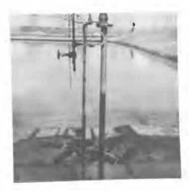
Figure 4. Bypass Line From Corrugated Plate Interceptor Hunt/Tuscaloosa
