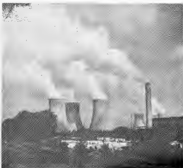
Figure 1. Sequence of photographs, about 5 seconds apart, of the cooling towers at Didcot, England. Flow separation is especially evident in the discharge from the middle tower.
