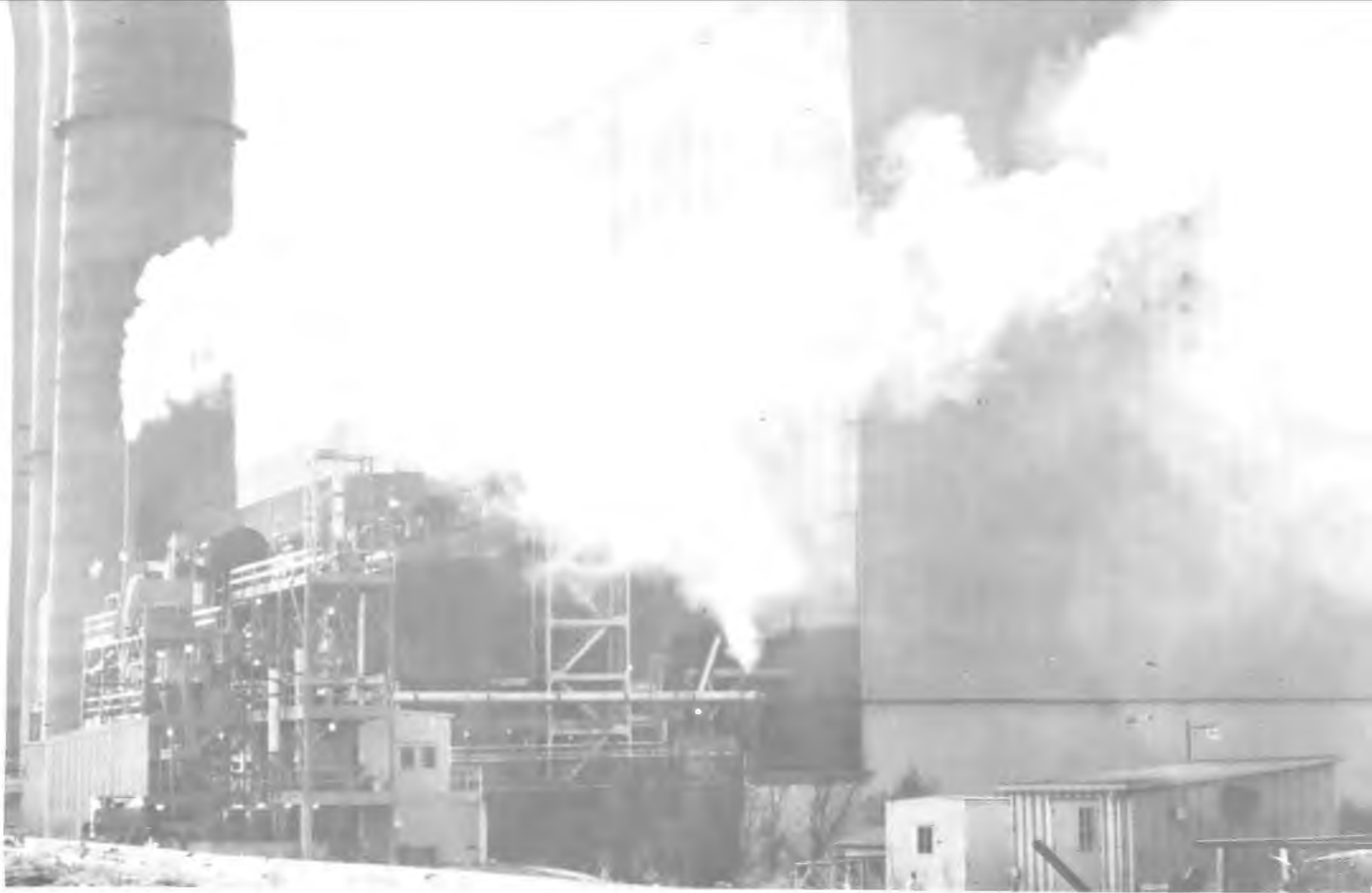
Figure 3. Typical plume during routine operation; high scrubber liquor concentration ( C = 10 ); no reheat.
