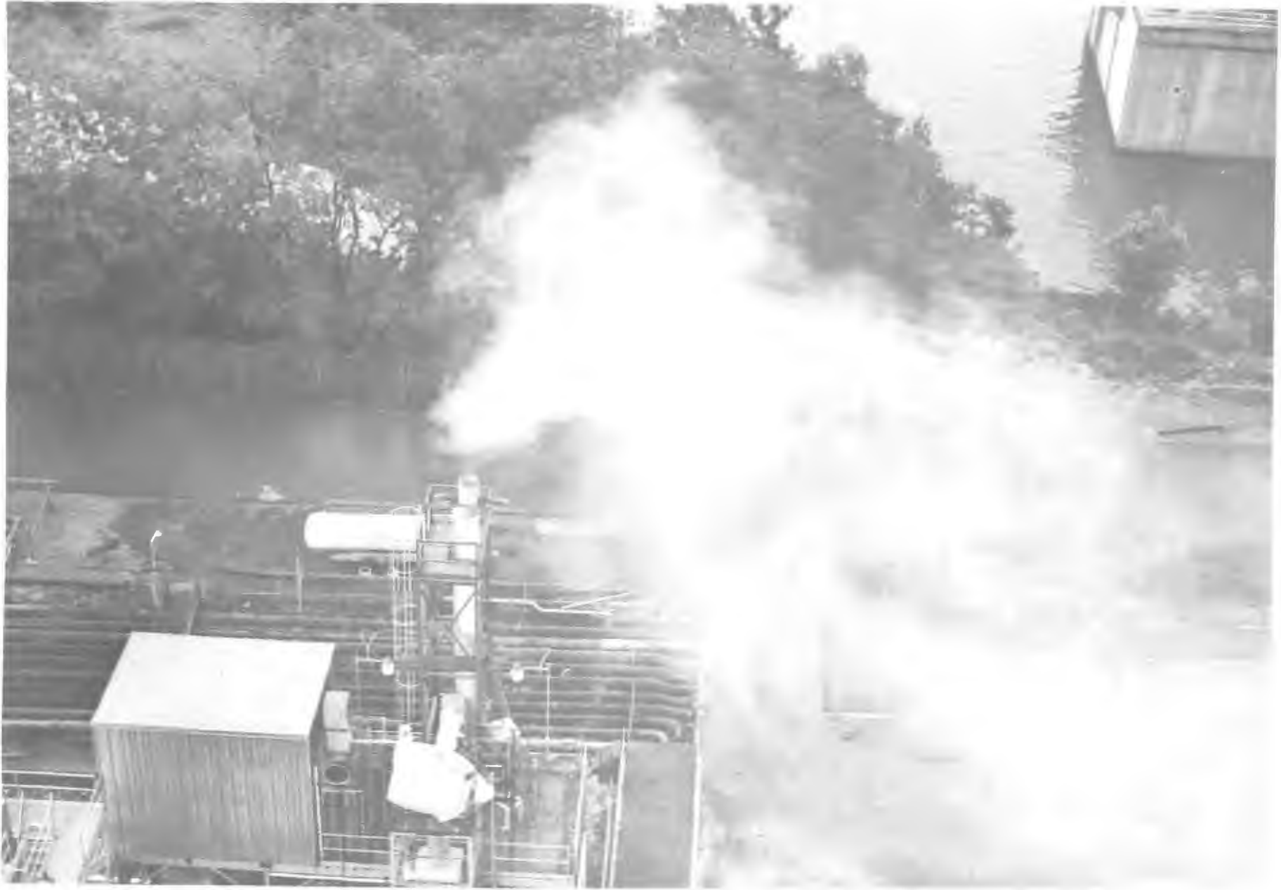
Figure 15. Plume reforming downwind of stack.
