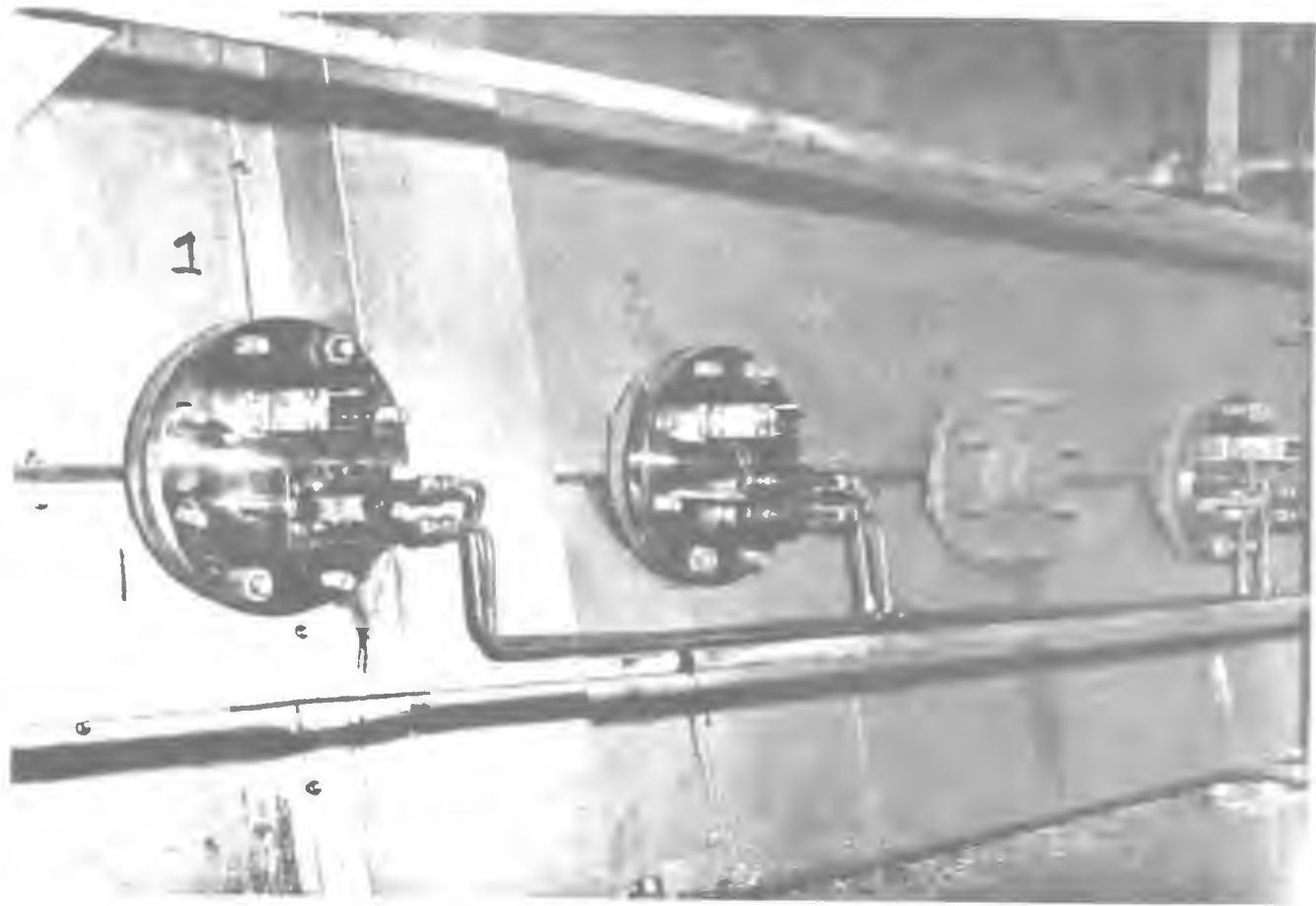
FIGURE 32 6 INCH PORTS SHOWING MANIFOLDING OF RAKES
