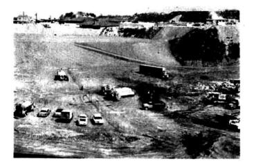
by road grades, traffic, and weather conditions. Time—travel studies are made by actually driving the loaded refuse vehicle from the collection area to each proposed site.
