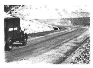
will have traction. Grades in excess of 7 percent are difficult for loaded trucks.
