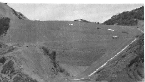
Cover is important, because more than any other single factor it makes a sanitary landfill nuisance free. It keeps rodents out and odors in. It prevents fires and keeps papers from scattering in the wind. Each day's refuse is sealed in an earthen cell.
