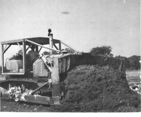
The crawler tractor equipped with a bulldozer blade is the mainstay of sanitary landfill equipment. Los Angeles uses them for compacting, having found that special compacting equipment does not appreciably increase the in-place density of solid wastes.
