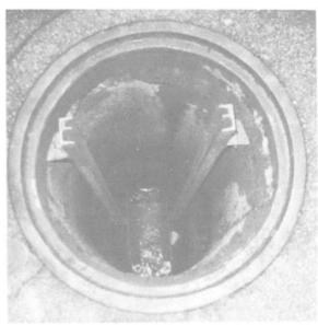
Figure 5. INSTALLATION OF SHEET METAL CHANNEL AND GUIDES FOR SAMPLING EQUIPMENT
