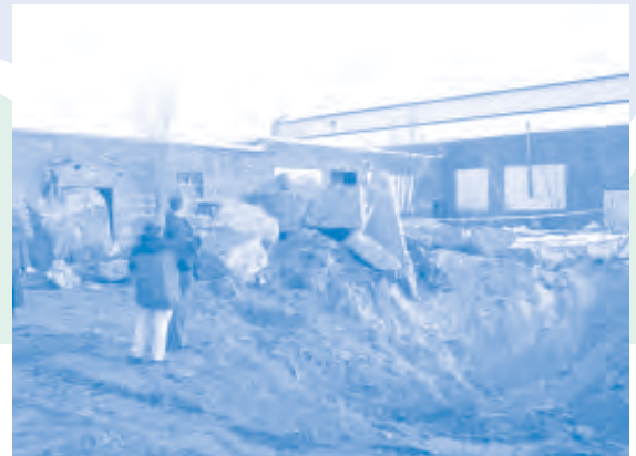
During demolition of parts of main building
