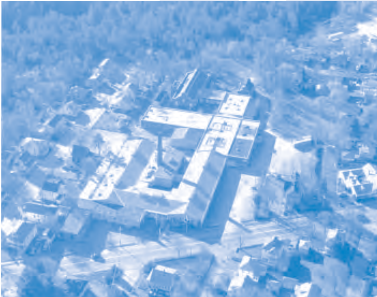
Aerial view of Whitney Screw complex and property
