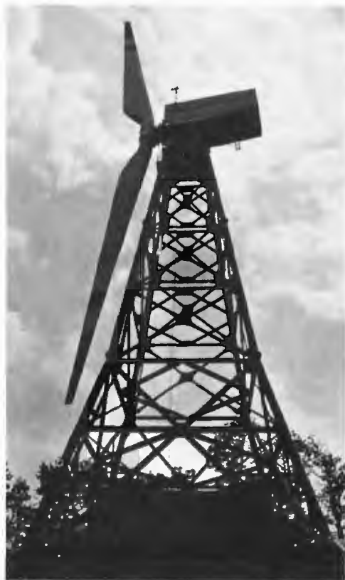
Wind turbine at Boone, N.C. generates 2,000 kilowatts for local power grid.
