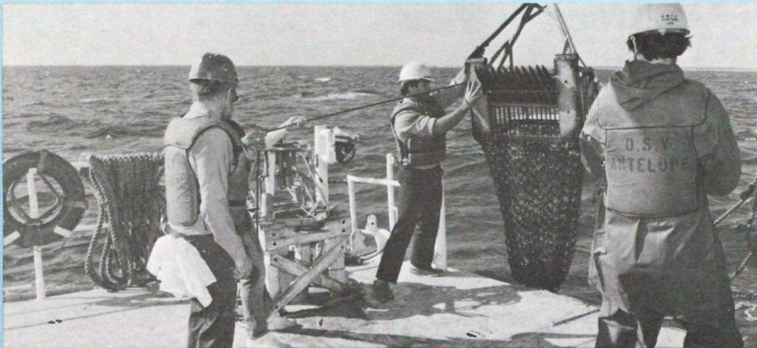
Crew members lower a bottom dredge, which rakes through sediment to collect bottom-dwelling organisms.
