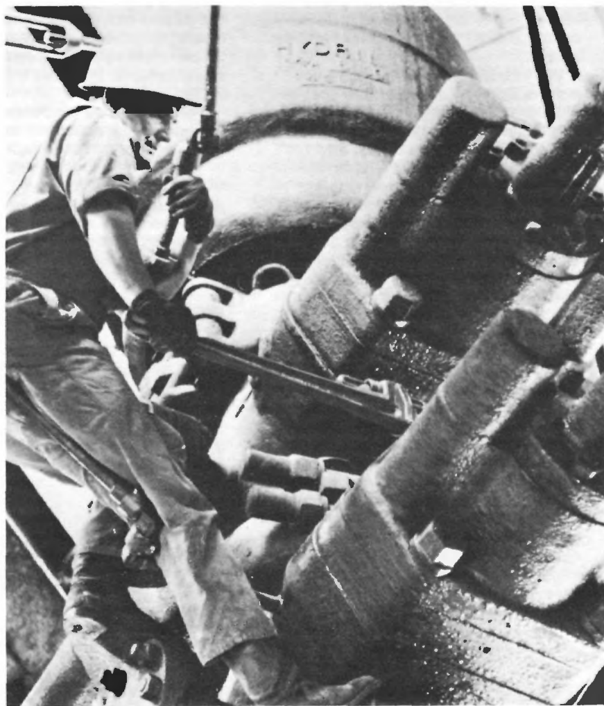
Workman prepares a blowout preventer for installation on an oil well being drilled off the Louisiana coast.
