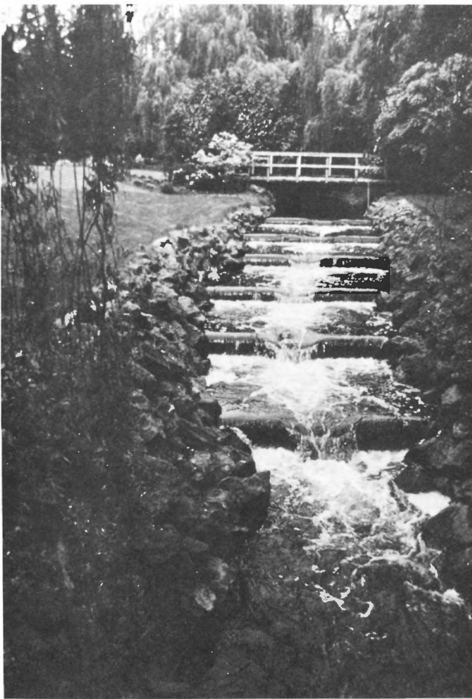
A fish ladder in Kelsey Creek in Bellevue, WA. The stream also doubles as part of the city's storm water drainage system. The city has tried to maximize the use of natural streams for its drainage system, while maintaining their natural beauty and reducing nonpoint source pollution.
