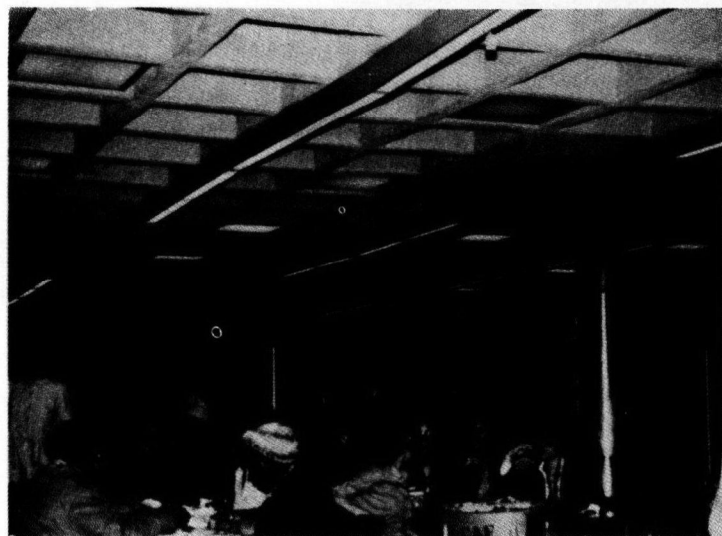
Cafeteria With Friable Material Ceiling Surface
