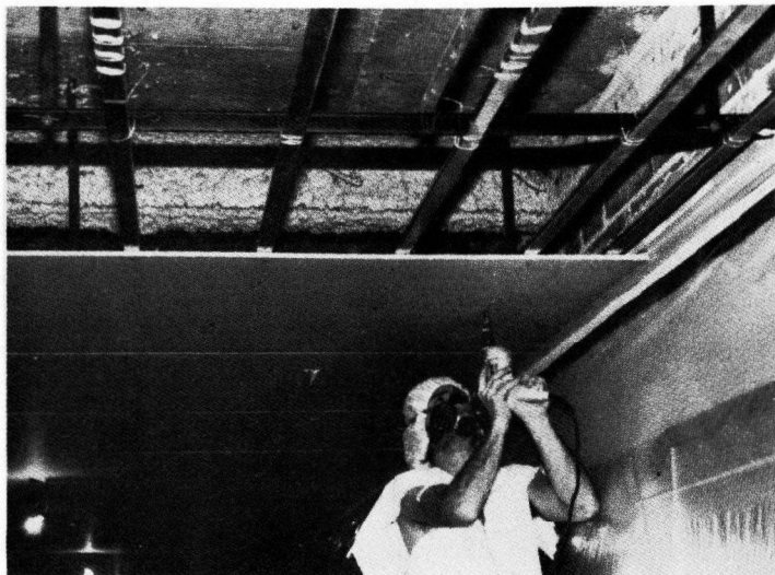
Constructing a Suspended Ceiling Barrier
