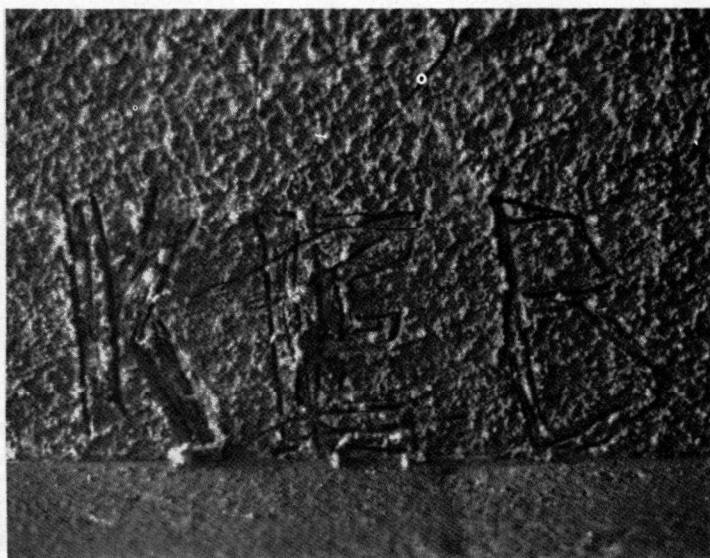
Friable Material That Has Been Scraped
