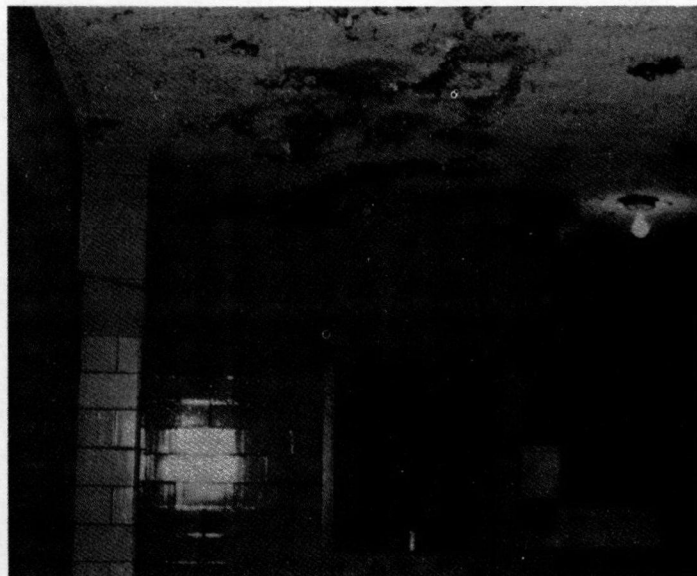
Friable Material Showing Water Damage
