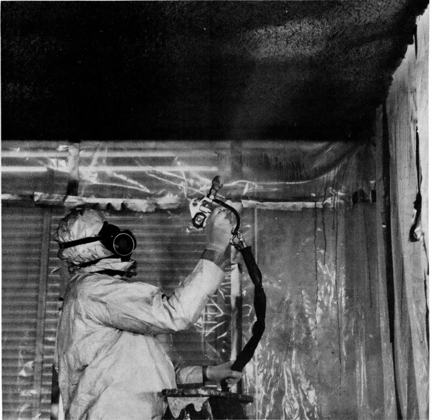
Encapsulation of a Ceiling Surface
