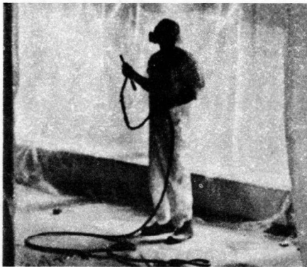
Ceiling asbestos wetted to decrease airborne fibers during removal process.
