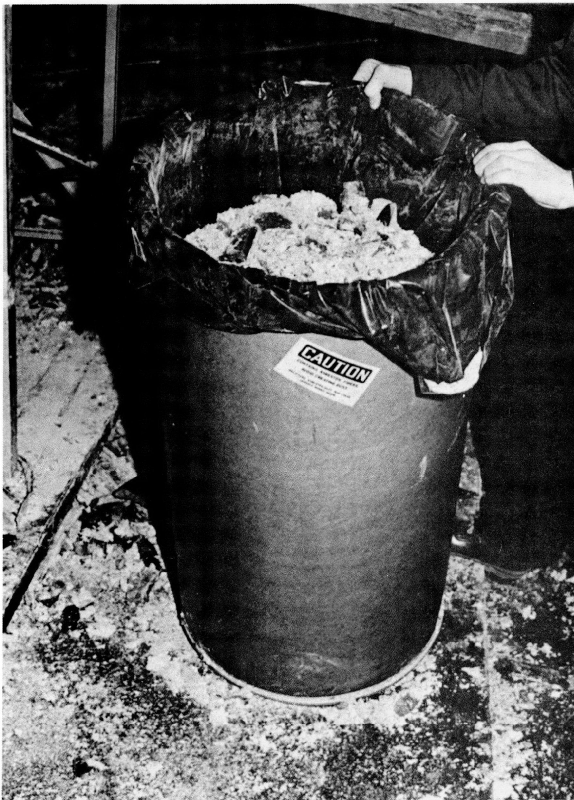
Figure E-2. Drum with 6-mil plastic liner to contain removed debris.
