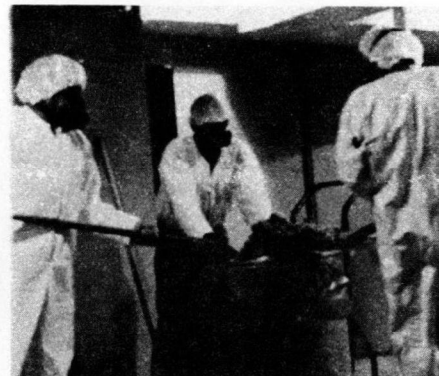
Asbestos material being loaded in approved containers.
