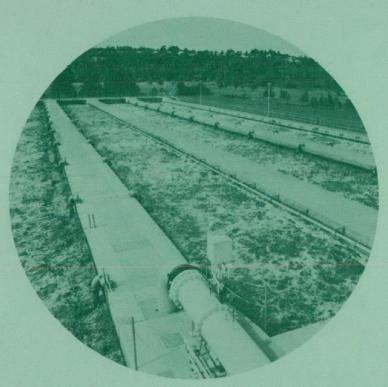
More than 95 percent of the suspended solids from raw sewage are removed by the treatment plant at Renton.
