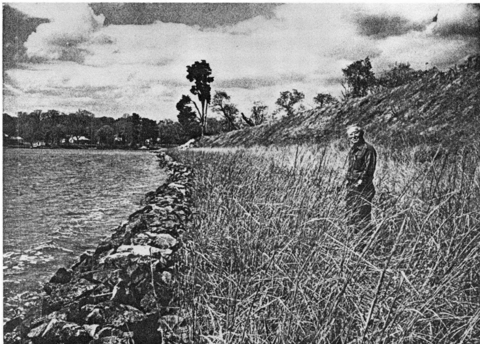
Figure 6. Stabilized Shoreline Using Sill and Marsh Grass.
