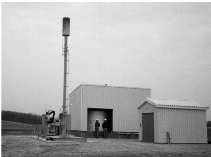
Figure 5-6. Skid-Mounted Open Flare and Blower Station.
