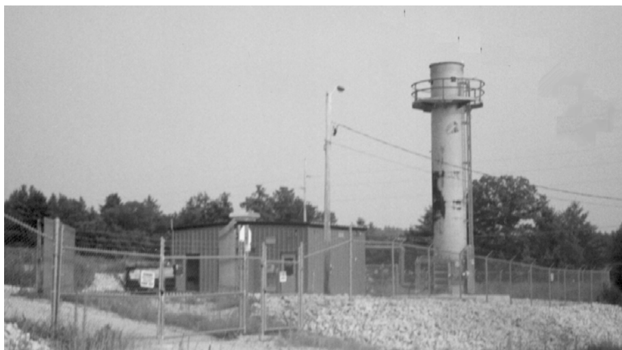
Figure 5-7. Enclosed Ground Flare and Blower Station.
