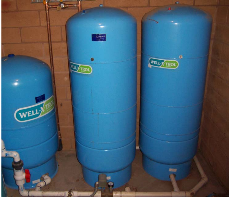
Figure 4-2. Pre-Existing Pressure Tanks
