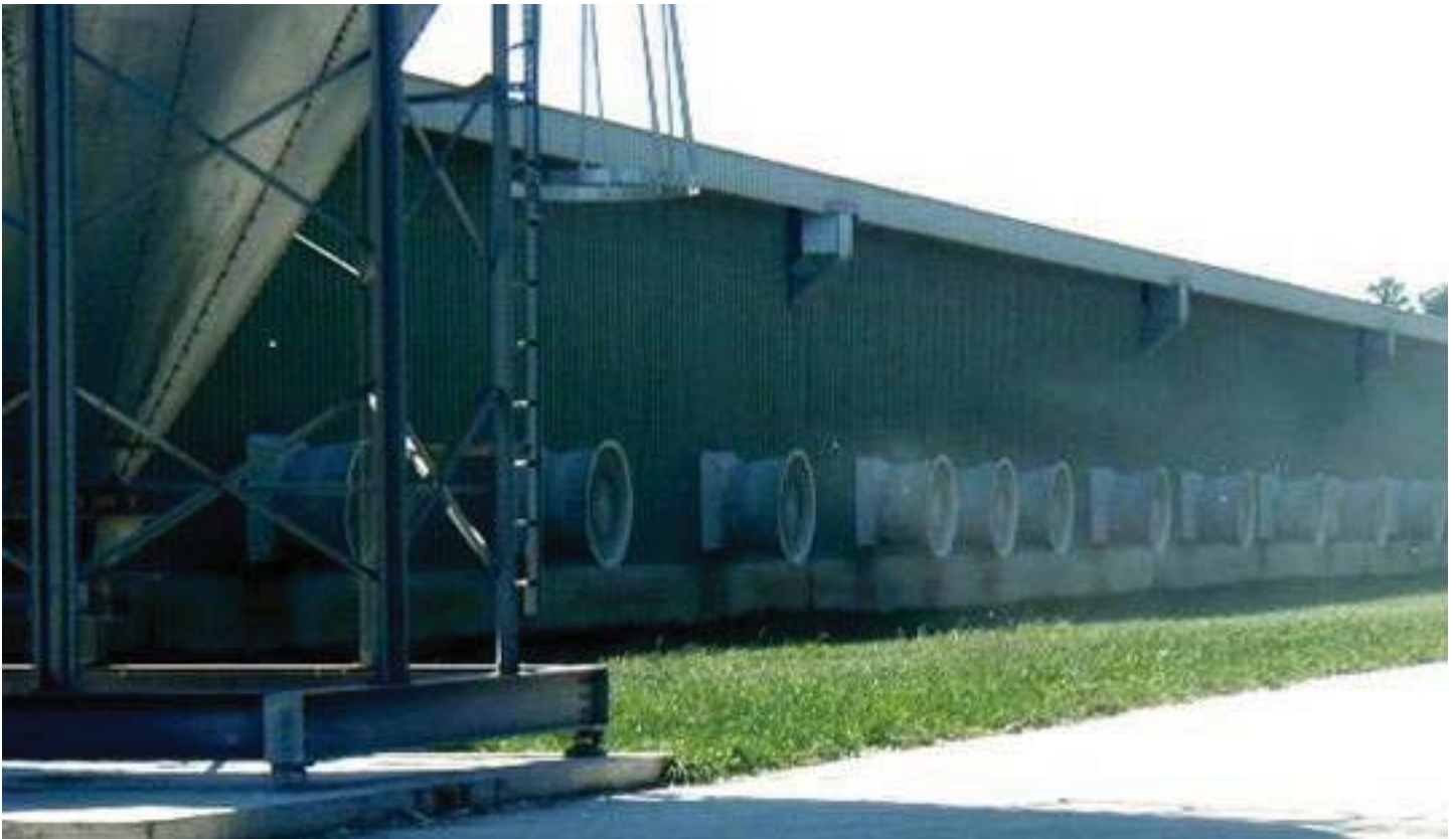
Barn exhaust fans generate visible air emission from an egg-laying facility
