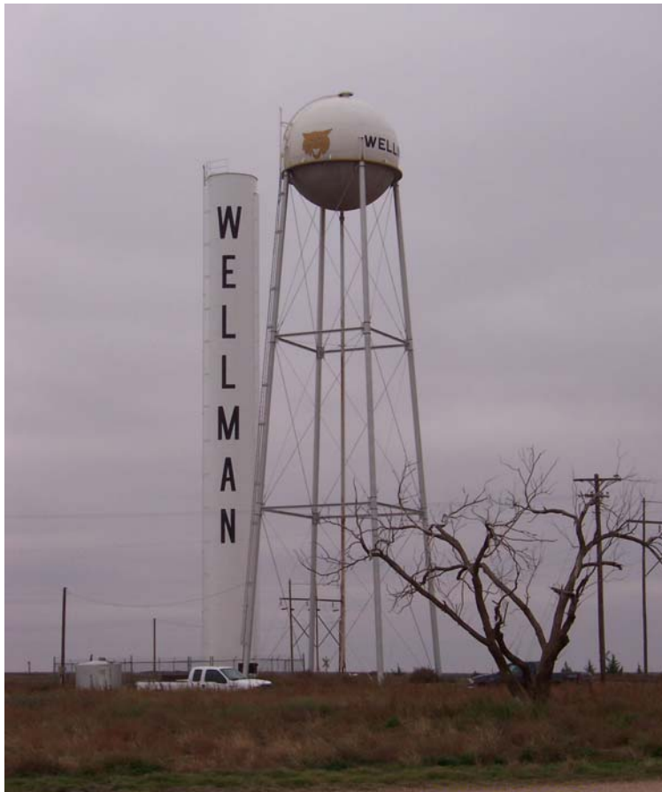
Figure 4-1. Water Tower and Chlorination Shed (Small Grey Structure Left of Truck)
