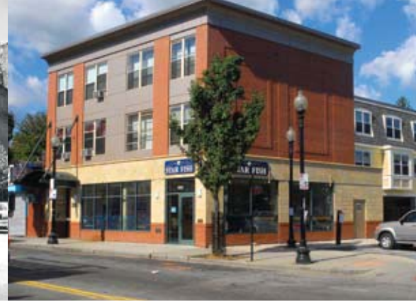
The redevelopment of Egleston Crossing used green design and energy-efficient materials, which reduce utility costs for residents.
