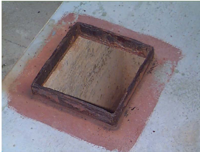
Exhibit 2.2 Raised Sill Appropriate for a Hatch
