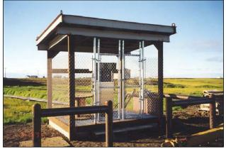
Figure 3-2. Fencing around a dispenser pump.
