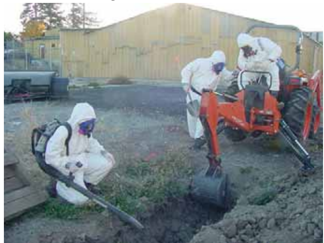
Figure 9. Task Based Monitoring in Phase III Excavation at Area A/B
