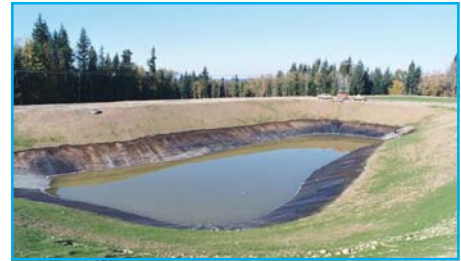
A sedimentation basin for storm water control.
