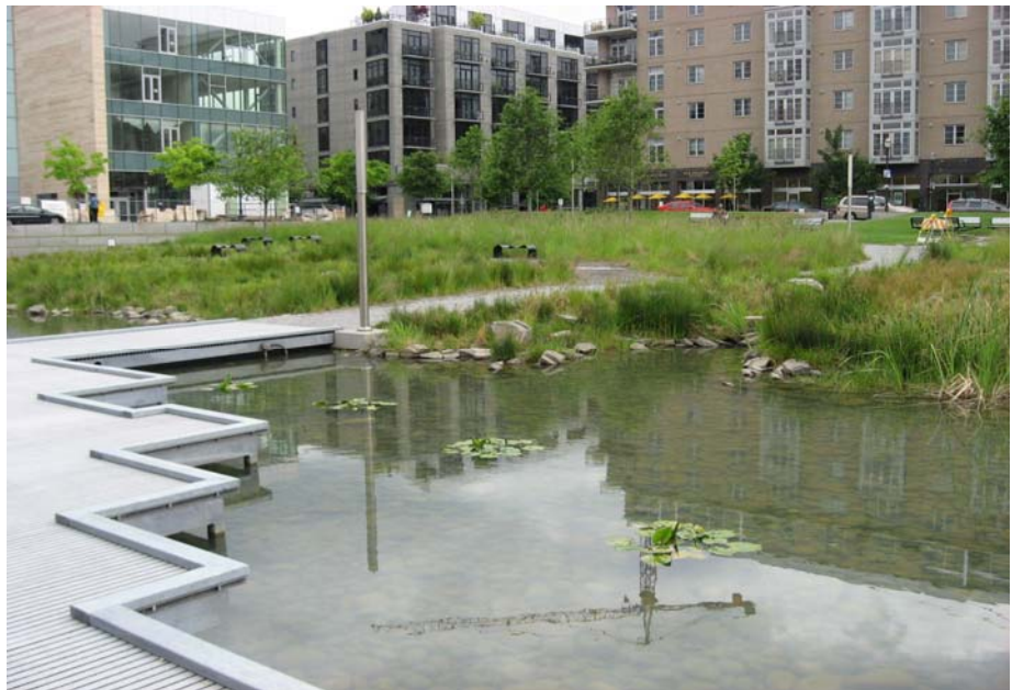
Tanner Springs Park in Portland, Oregon includes a constructed wetland for managing runoff from nearby buildings
