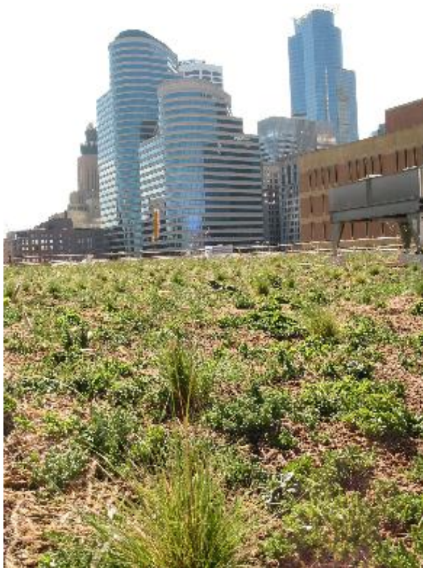
Minneapolis Central Library Green Roof. Image courtesy The Kestrel Design Group, Inc.
