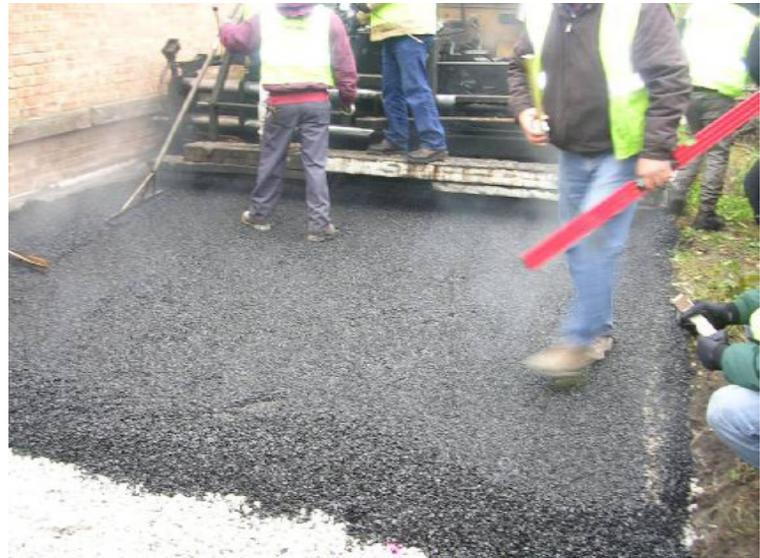
**Figure 9: Permeable Asphalt Installation Using Ground Tire Rubber.**
