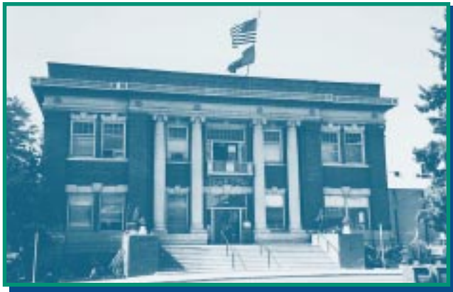
Klamath Falls City Hall uses geothermal district heating.
