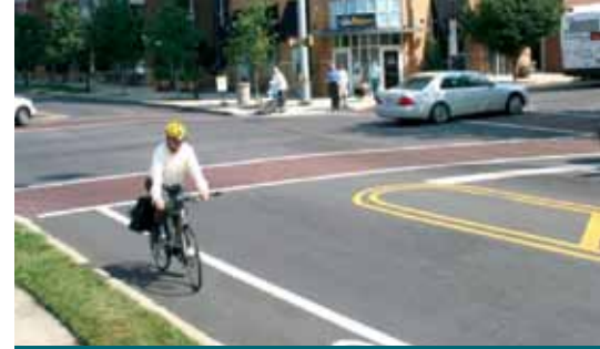
East Boulevard was a four-lane, undivided street carrying more than 20,000 vehicles a day through the heart of Dilworth, a historic neighborhood with multiple land uses in close proximity. The street was successfully converted to three lanes with bicycle lanes and pedestrian refuge islands.
