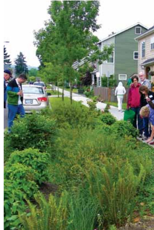
Rain gardens, such as these, effectively treat the New Columbia neighborhoods stormwater runoff, while also creating lovely public spaces.
