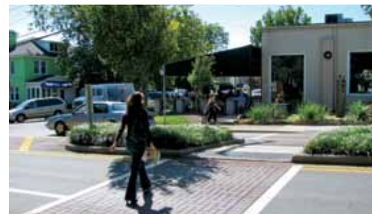
Elizabeth Avenue connects uptown Charlotte to one of the city's historic suburbs. In a collaborative effort, Elizabeth Avenue was reconstructed to be more pedestrian friendly with more landscaping and improved crosswalks.
