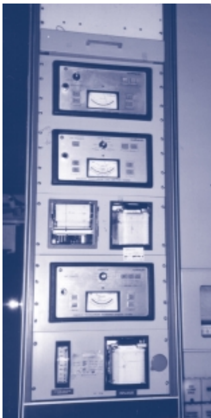
\text{SO}_2 and \text{NO}_x CEM machine.
