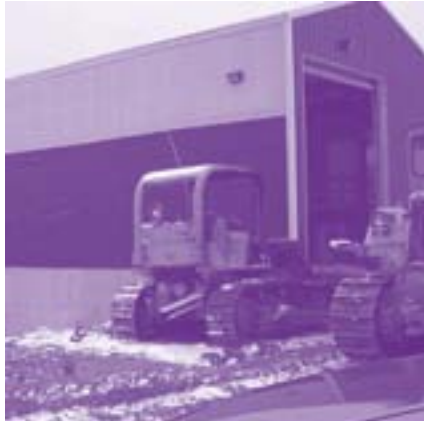
Turtle Mountain's new transfer station.
