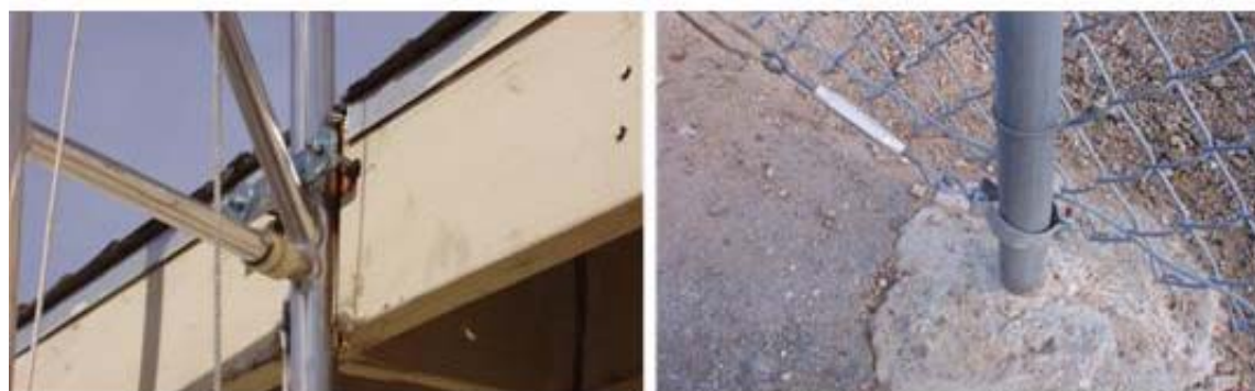
Figure 1.7 (a) Fascia Board Support; (b) Fence Post Guy Wire Anchor
