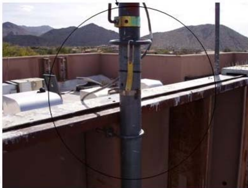
Figure 1.9 (a) Metal Wall Support—Telescopic Tower (Expanded View); (b) Metal Wall Support—Telescopic Tower (Close-Up View)
