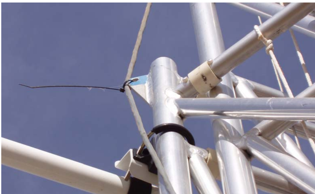
Figure 1.14 Wiring on a Crank-Down Tower
