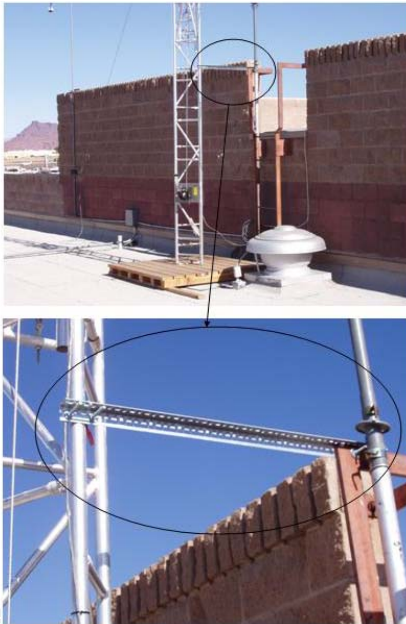
Figure 1.8 (a) Angle Iron Support—Expanded View; (b) Angle Iron Support—Close-Up View
