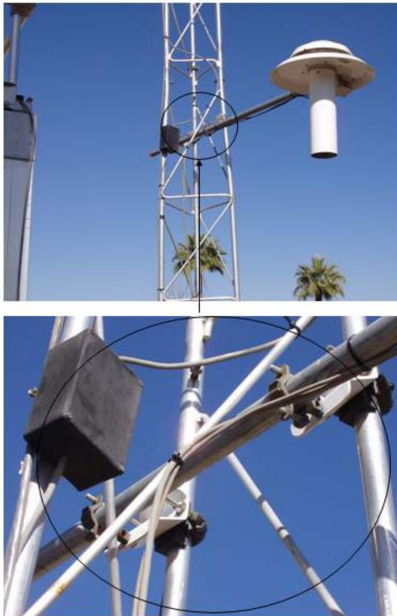
Figure 1.13 Temperature Cable Installation and Expanded/Close-Up Views
