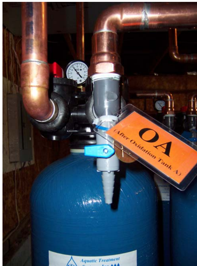
Figure 4-6. Close-Up View of a Sample Tap (OA), a Pressure Gauge, and Copper Piping at Head of a Column
