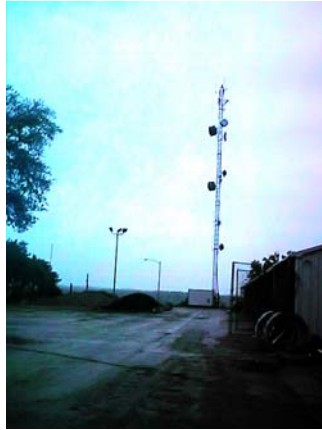
Figure 5-3. Picture of a radio transmission tower.
