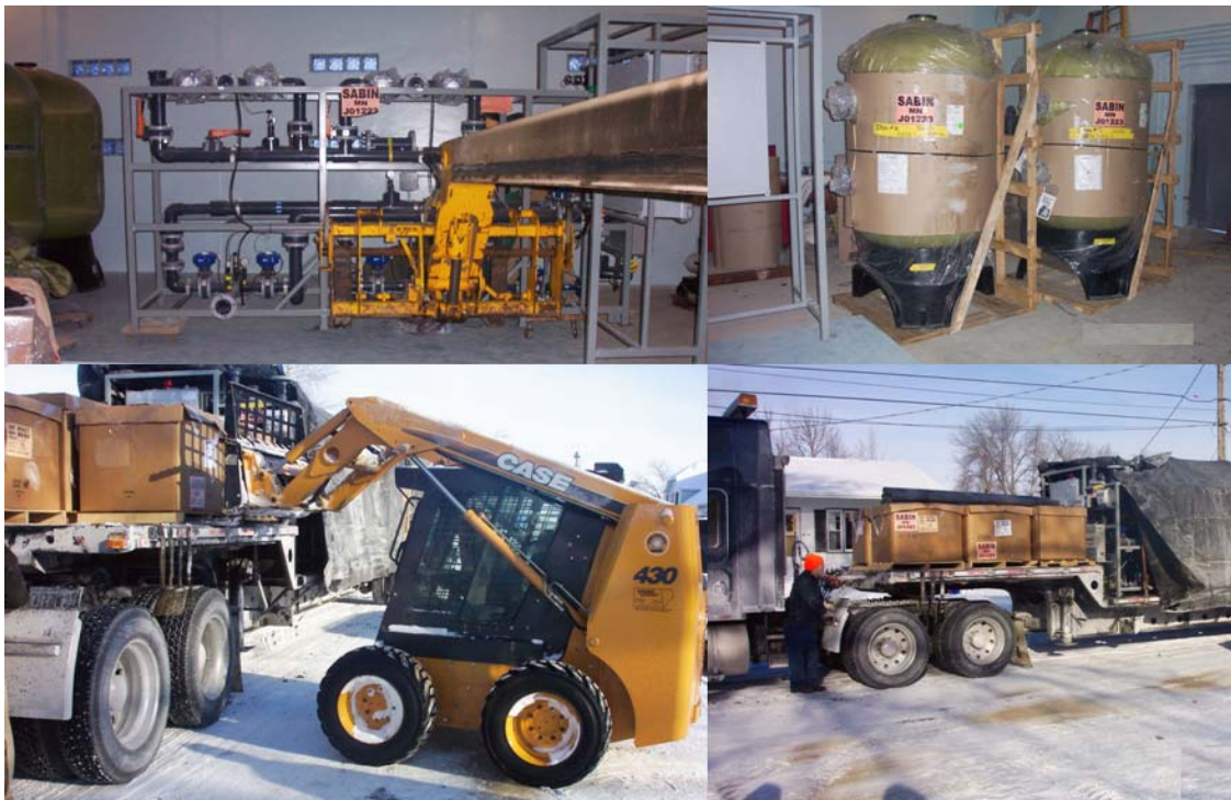
Figure 4-7. Delivery and Off-Loading of Macrolite ® Treatment System Equipment
