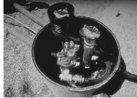
Open manway showing catch basin and pressurized piping (without the line leak detector yet installed).
