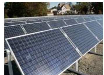
Top: Tracking PV panels follow the sun to allow for increased solar capture. Bottom: Fixed axis PV panels aligned to be south facing.
