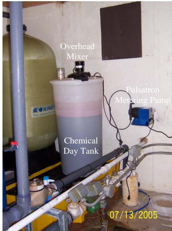
**Figure 4-5. KMnO<sub>4</sub> Feed System**
