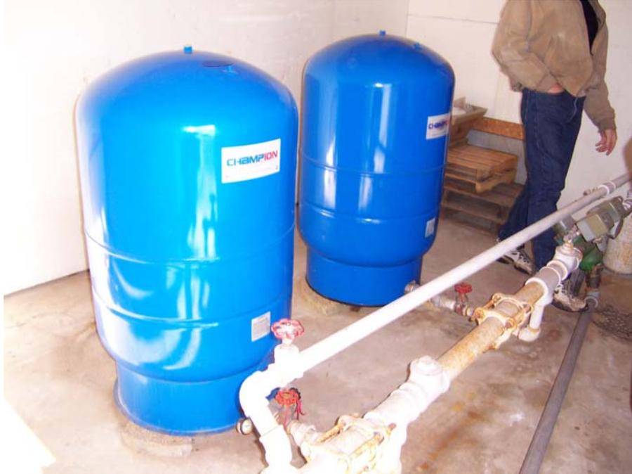
**Figure 4-2. Existing Well Piping and Pressure Tanks at BSLMHP, MN Site**
