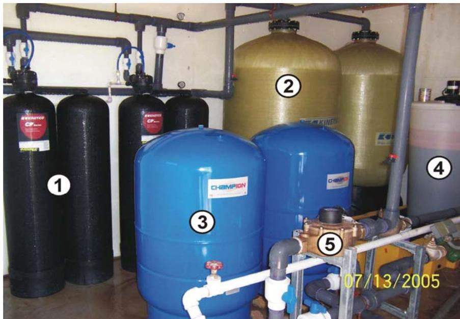
**Figure 4-4. Photograph of Macrolite® Pressure Filtration System**
