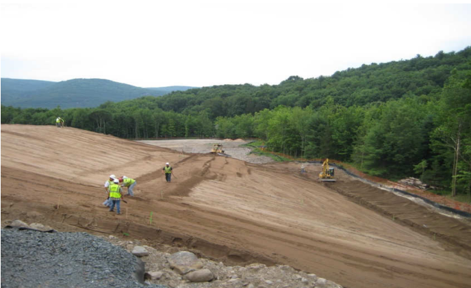
Contouring for landfill cover at Ellenville Scrap Iron and Metal, Ellenville, NY
