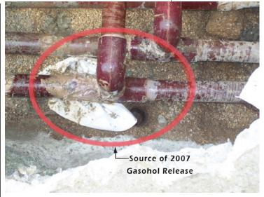
**FIGURE 1.** "T" fitting under the dispenser where 2007 release occurred.
