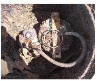
An ATG probe area from a 2010 inspection at an E10 facility. Notice the extreme corrosion throughout.
