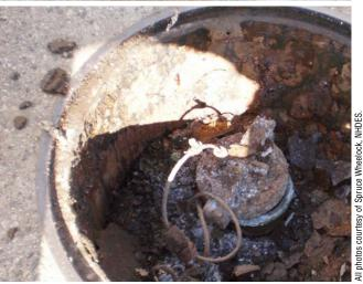
Top: Typical ATG riser installation surrounded by the tank backfill. Overfill events can leak from such unprotected risers and spill directly into the tank backfill. Such releases can be prevented by locating all risers within a collared sump.
