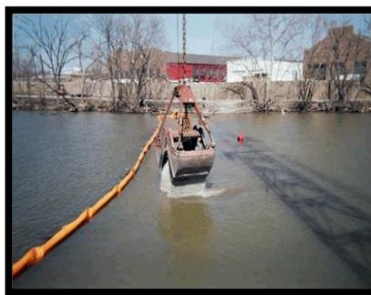
Applying capping materials with a clamshell bucket
