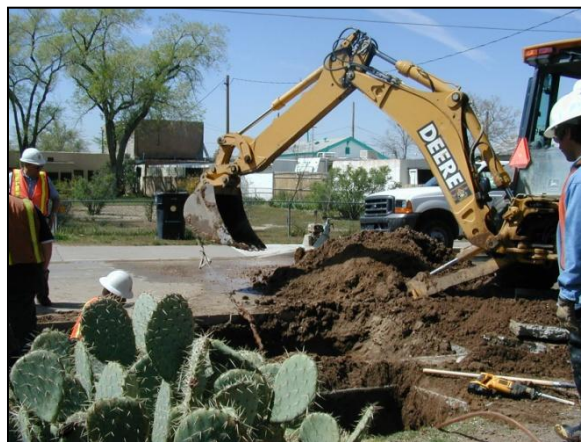
Digging up leaking water lines in Albuquerque, NM
