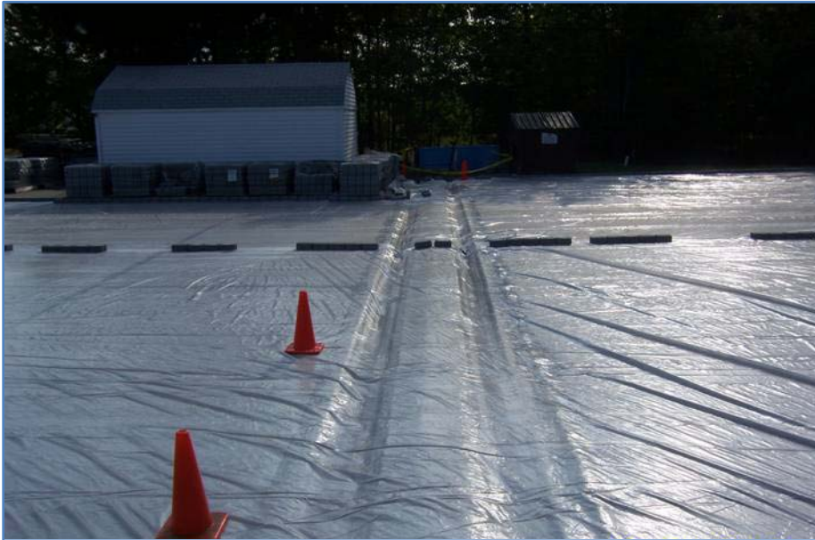
Figure 6. Parking lot central drains covered in plastic for rainwater collection.
