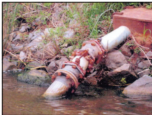
This pipe is the first underwater extension of Arkla's river outfall. The underwater piping prevented the detection of the illegal river discharges.
