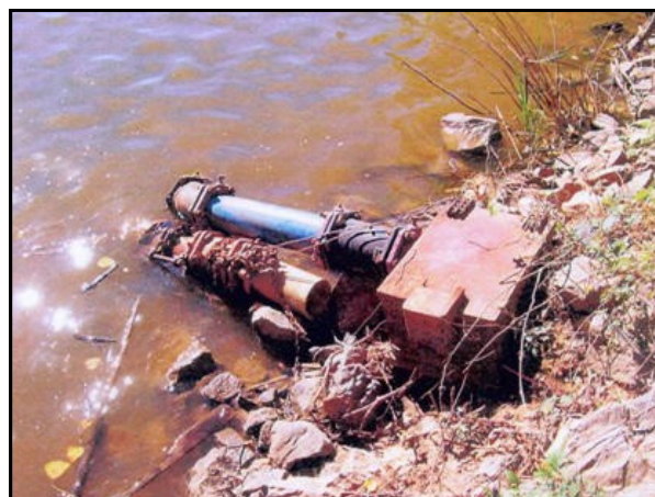
This is the second underwater extension of Arkla's river outfall. The blue piping was added in Sept 2007, shortly before the welded bypass was added at the facility. The piping was added to hide the illegal river discharges.
