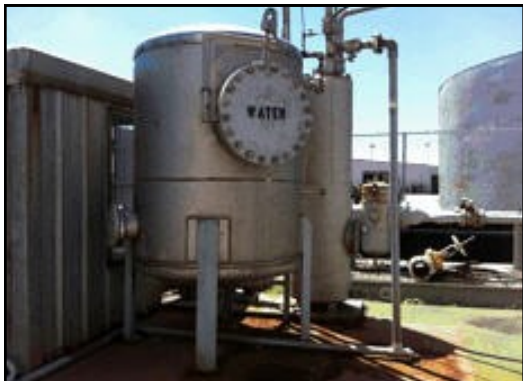
Wastewater holding tank that, at times, would bypass treatment and discharge directly to the Intracoastal Waterway Canal.
