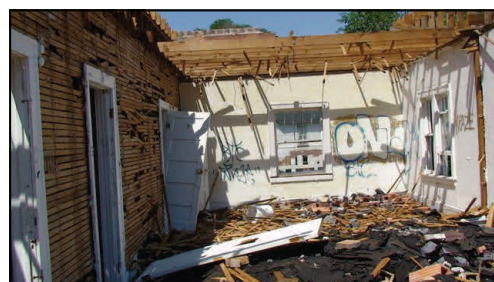
Pictures depicting demolition work that resulted in the release of asbestos
