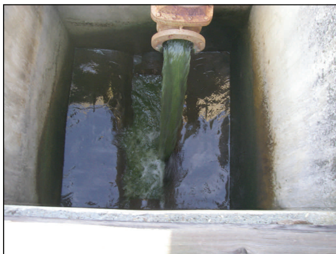
Wastewater influent pipe at Rising Sun Subdivision POTW
