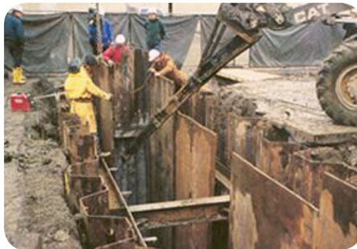
Construction of a PRB in Sunnyvale, CA
