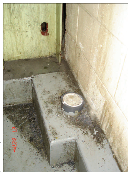
Cut illicit discharge pipe entering the floor drain
