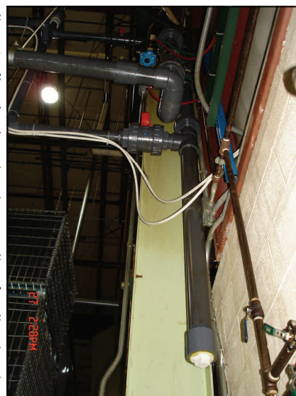
Cut illicit discharge pipe
