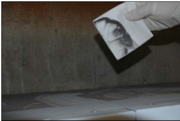
Figure 5 Equipment Room Locker Top Wipe Sample (11 µg PCBs)
