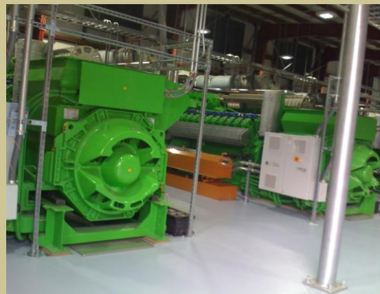
Methane gas generators at the Anchorage Regional Landfill Photo by the Author
