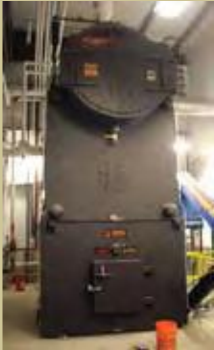
Wood chip burner in Tok Photo from Alaska Energy Authority 2011 Renewable Energy Atlas
