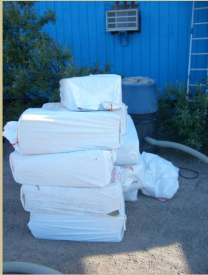
Cellulose insulation added to the village store in Anaktuvuk Pass to improve heating efficiency.
