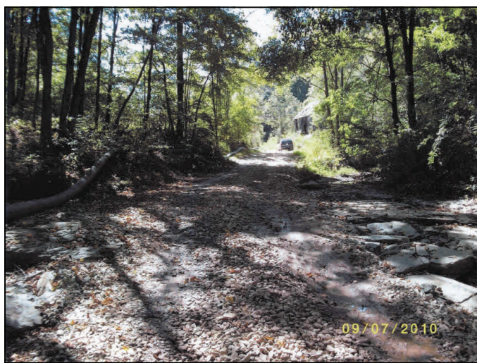
Blake Fork after having stone and gravel spread in the stream to create a roadway
