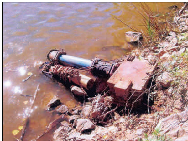
This is the second underwater extension of Arkla's river outfall. The blue piping was added in September 2007, shortly before the welded bypass was added at the facility. The piping was added to hide the illegal river discharges.
